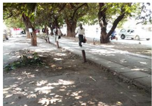
Above - Sections of the road island elsewhere which are not attended to
